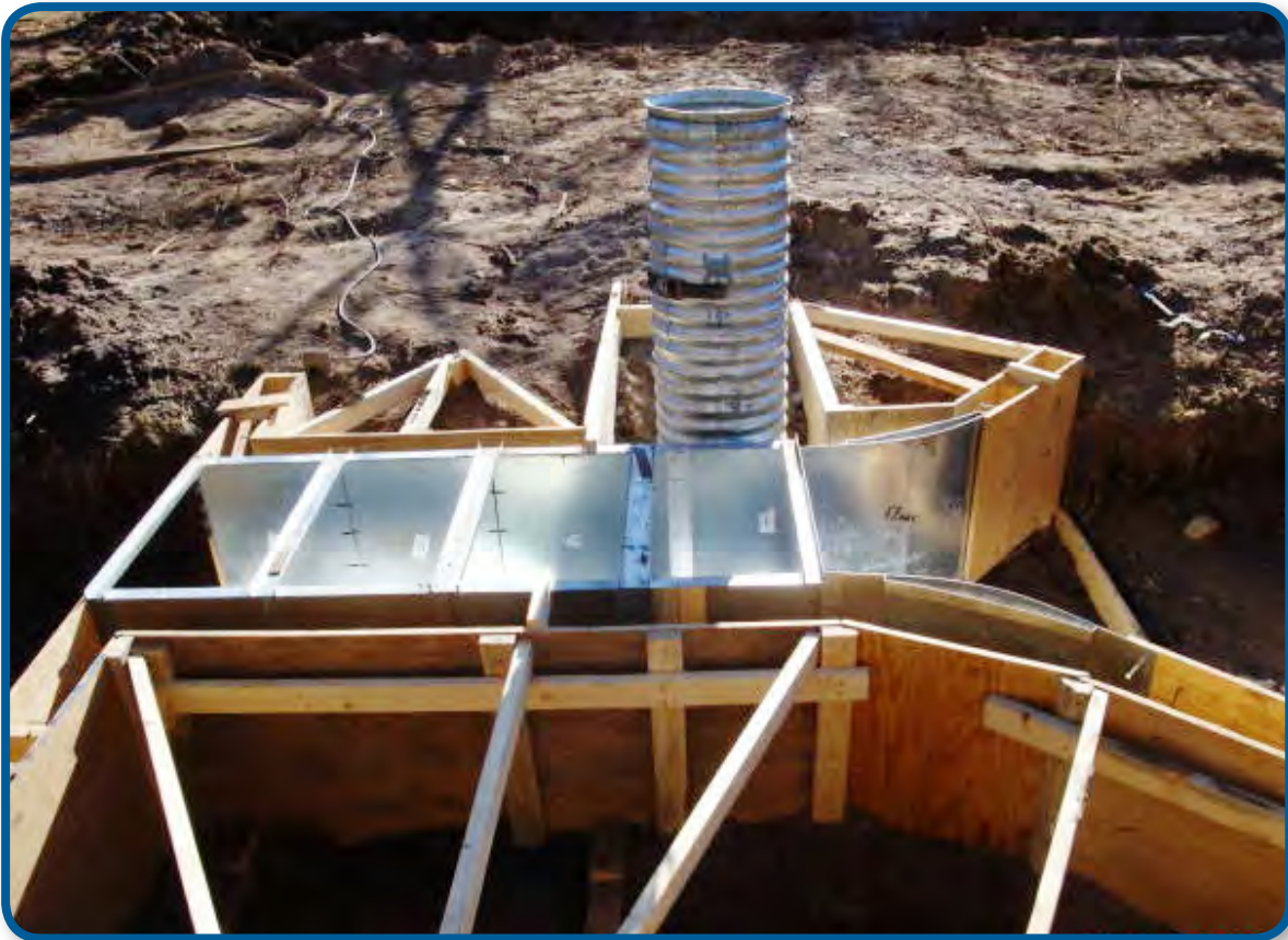
Framing Flume for Cement
