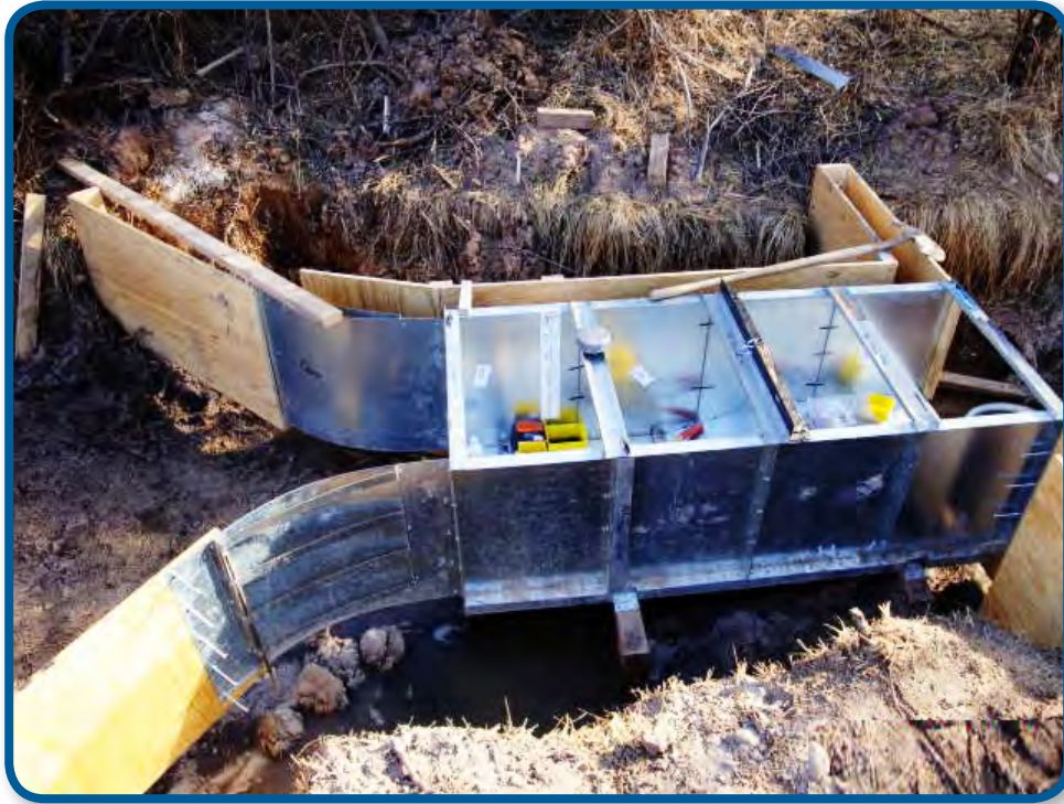
Framed Flume before Cement
