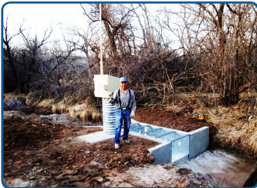
Completed Station Downstream
