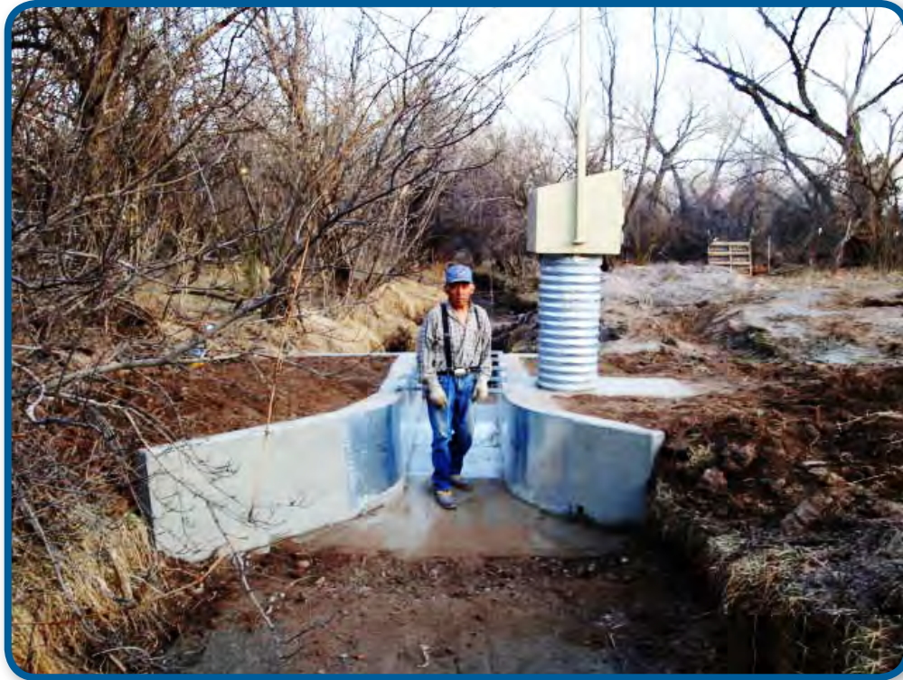
Completed Station Upstream
