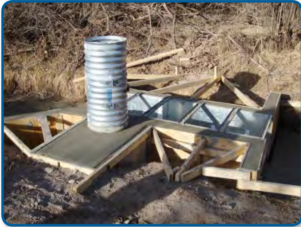
Framed Station after Cement
