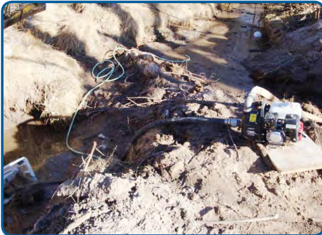
Bypass for Construction & Excavation
