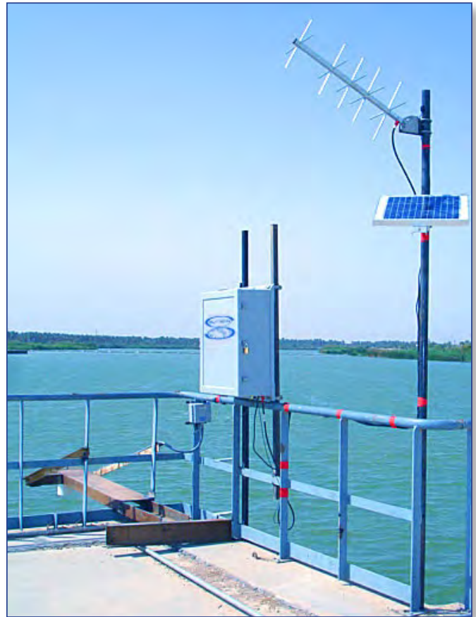
Sutron's Radar Gauging Station, Iraq
