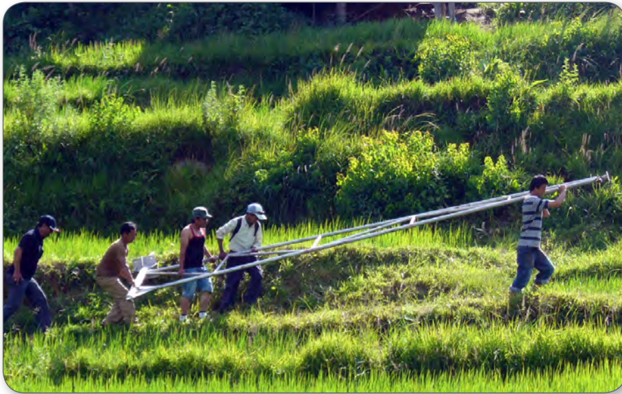
Yebessa AWLS Installation
