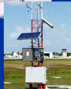
Sutron Installations - Albany, NY & the Cayman Islands Airport
