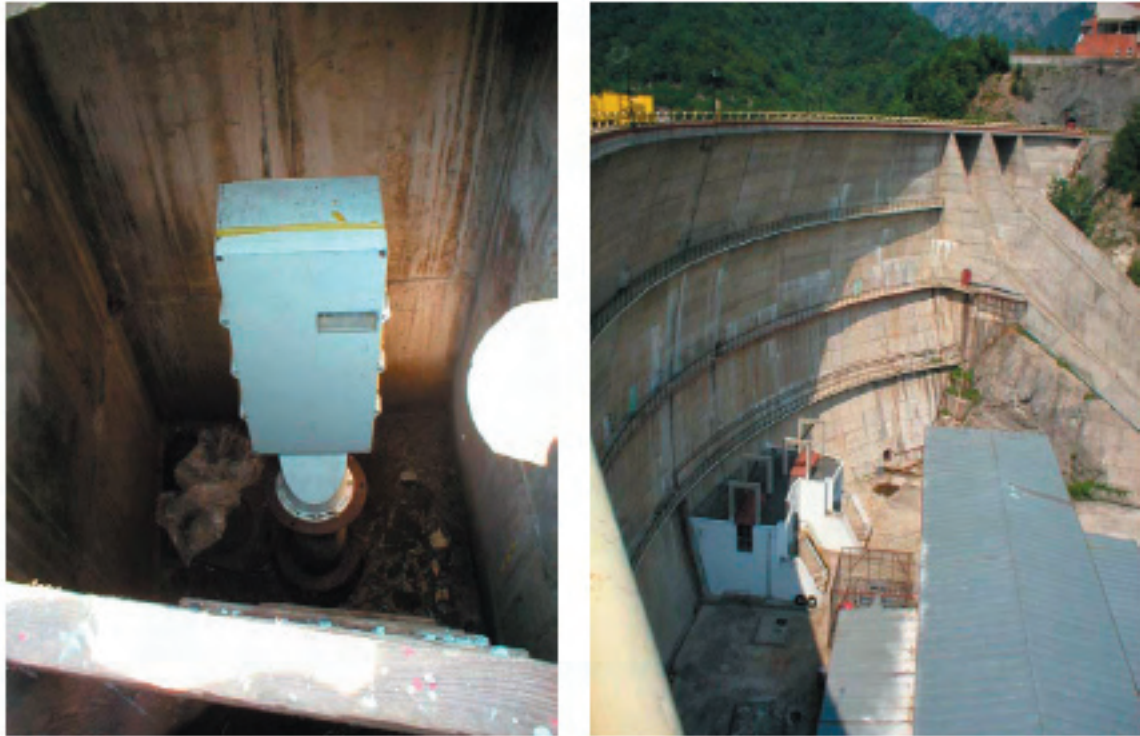
FIG. 2 – HERCULANE DAM (LEFT – THE OLD MEASURING SYSTEM; RIGHT – THE DAM. DOWN, THE VALVE).
