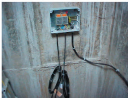
Fig. 3 - OVERVOLTAGE SENSORS PROTECTION
