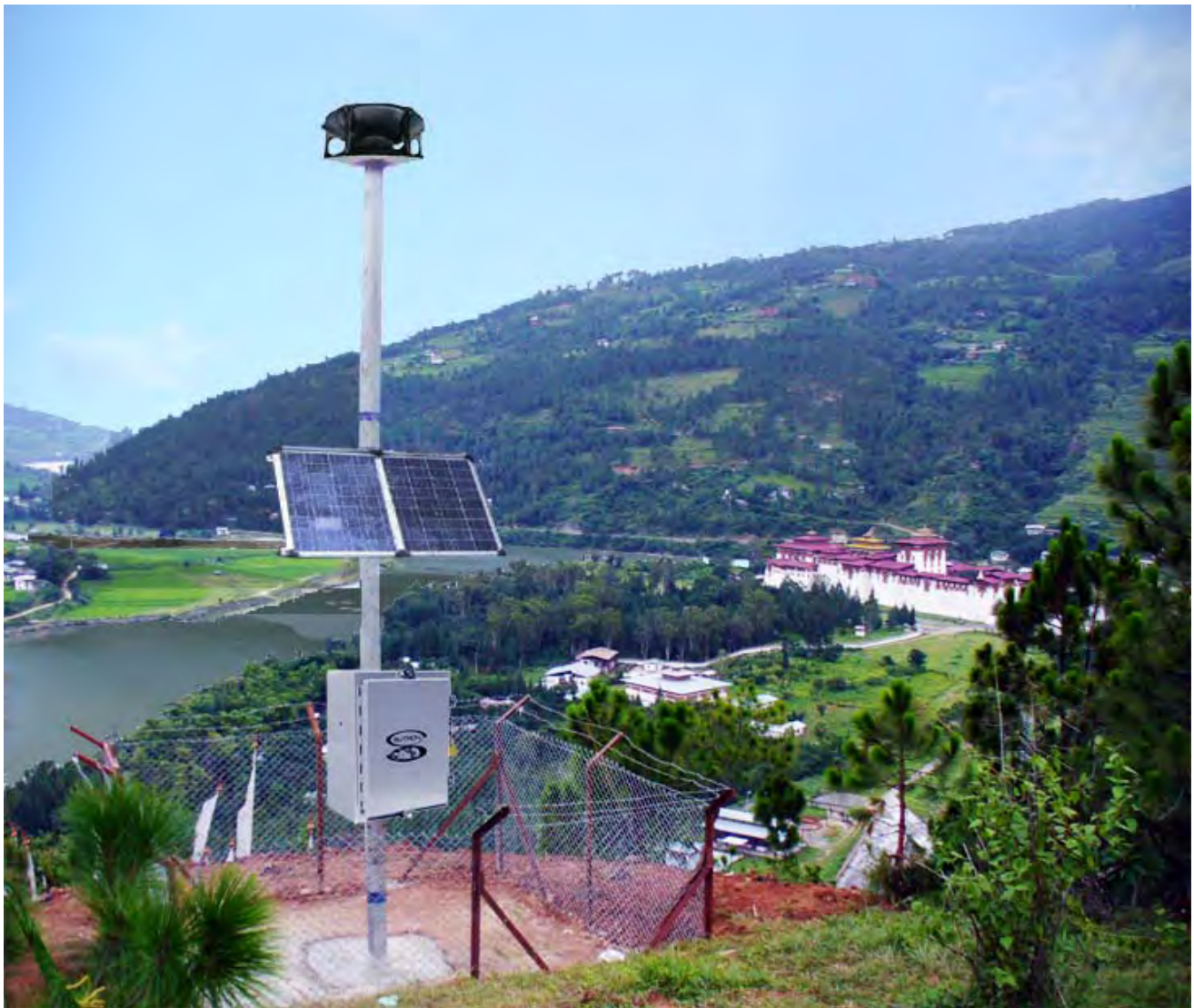
Siren Station Overlooking the Punakha Dzong, Bhutan
