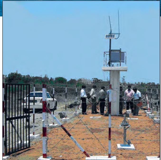
Equipment Installation at HFL
